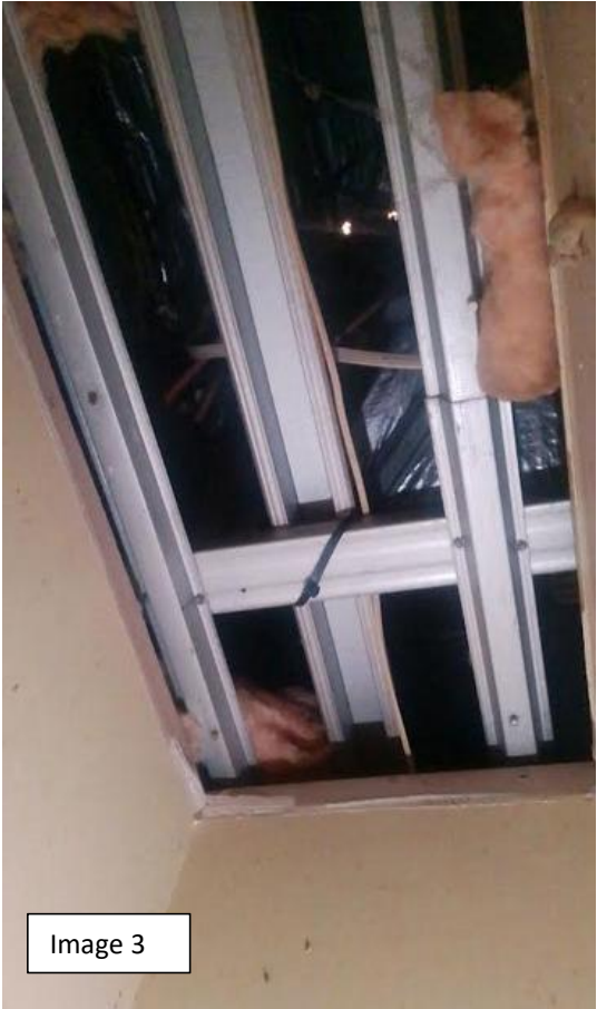
Ceiling collapse linen cupboard
